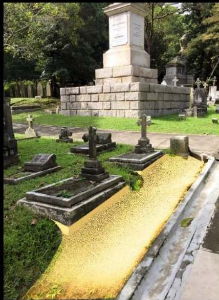
STEP 3 After the concrete settled, we will add the layer of soil.
