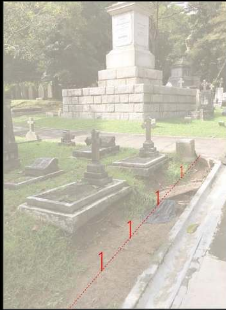
STEP 1 Planting steel picks to provide additional grip for the concrete.
